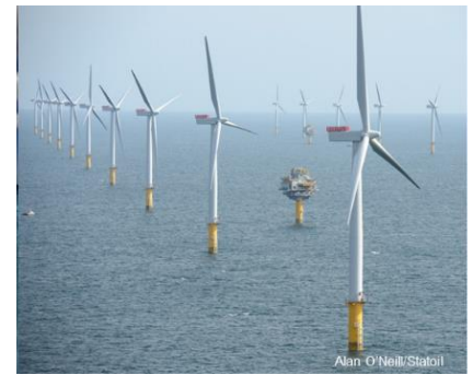
Utility scale Hywind 2020+
