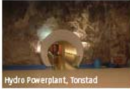
Hydro Powerplant, Tonstad
